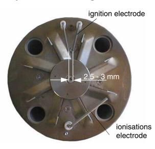
The ignition electrodes are preset at the factory.
