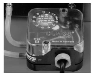
The air pressure switch is a differential pressure switch and monitors pressure at the forced-air burner.
