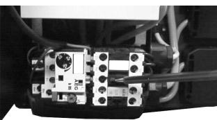
Once the connection to the electricity supply has been established, check the wiring and briefly actuate the motor contactor with an electrician's insulated screwdriver to check the direction of rotation of the burner motor.
