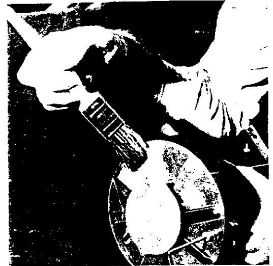
FIG.27 Cleaning of Air Diffuser and Gas Spreader
