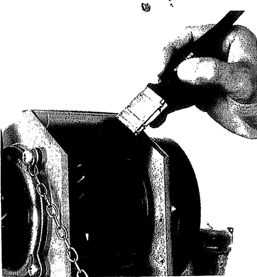
FIG.20 Cleaning combustion air fan
