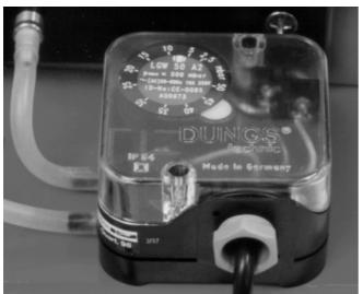
The air pressure switch is a differential pressure monitor and monitors pressure at the blower burner.
